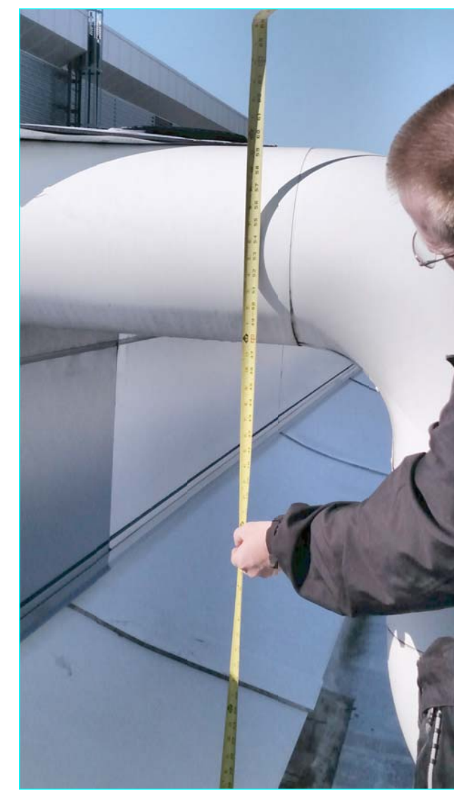
EXISTING CONDITION PHOTO 12 ROOF ACCESS LOCATION #7 SCALE: N.T.S.
