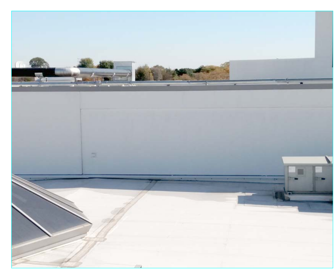
EXISTING CONDITION PHOTO 1 ROOF ACCESS LOCATION #1 SCALE: N.T.S.
