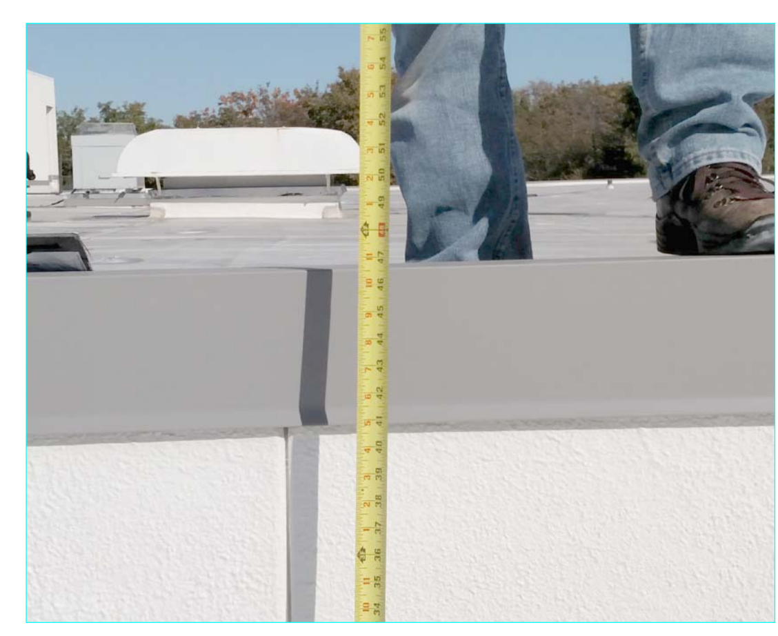
EXISTING CONDITION PHOTO 11 ROOF ACCESS LOCATION #3 SCALE: N.T.S.
