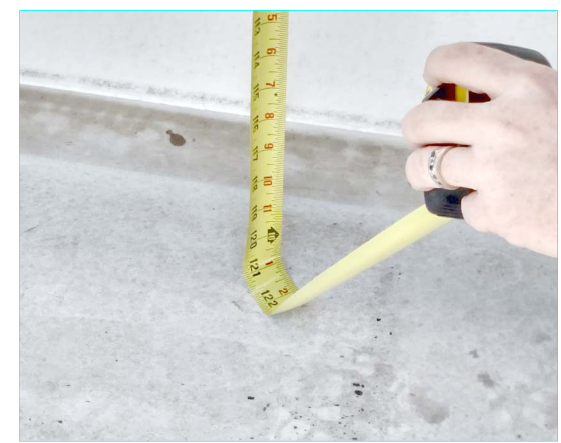
EXISTING CONDITION PHOTO 2 ROOF ACCESS LOCATION #1 SCALE: N.T.S.
