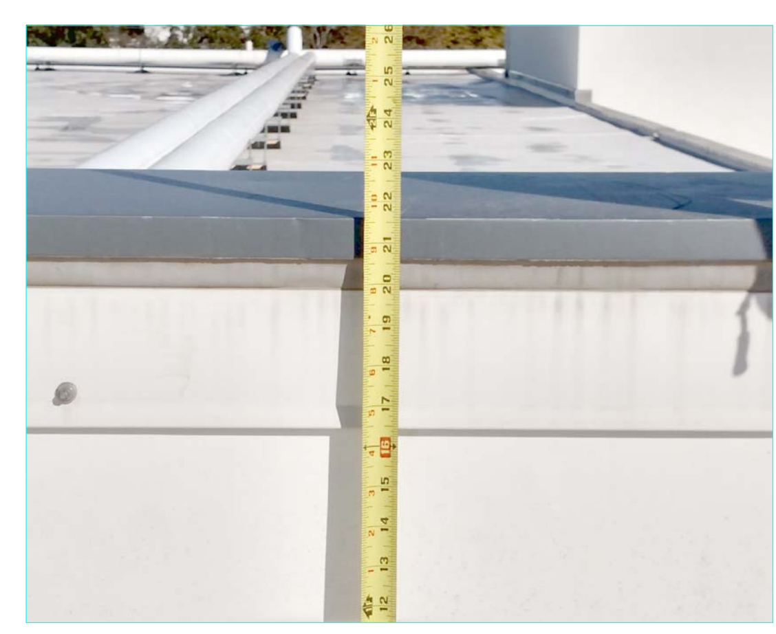
EXISTING CONDITION PHOTO 9 ROOF ACCESS LOCATION #7 SCALE: N.T.S.
