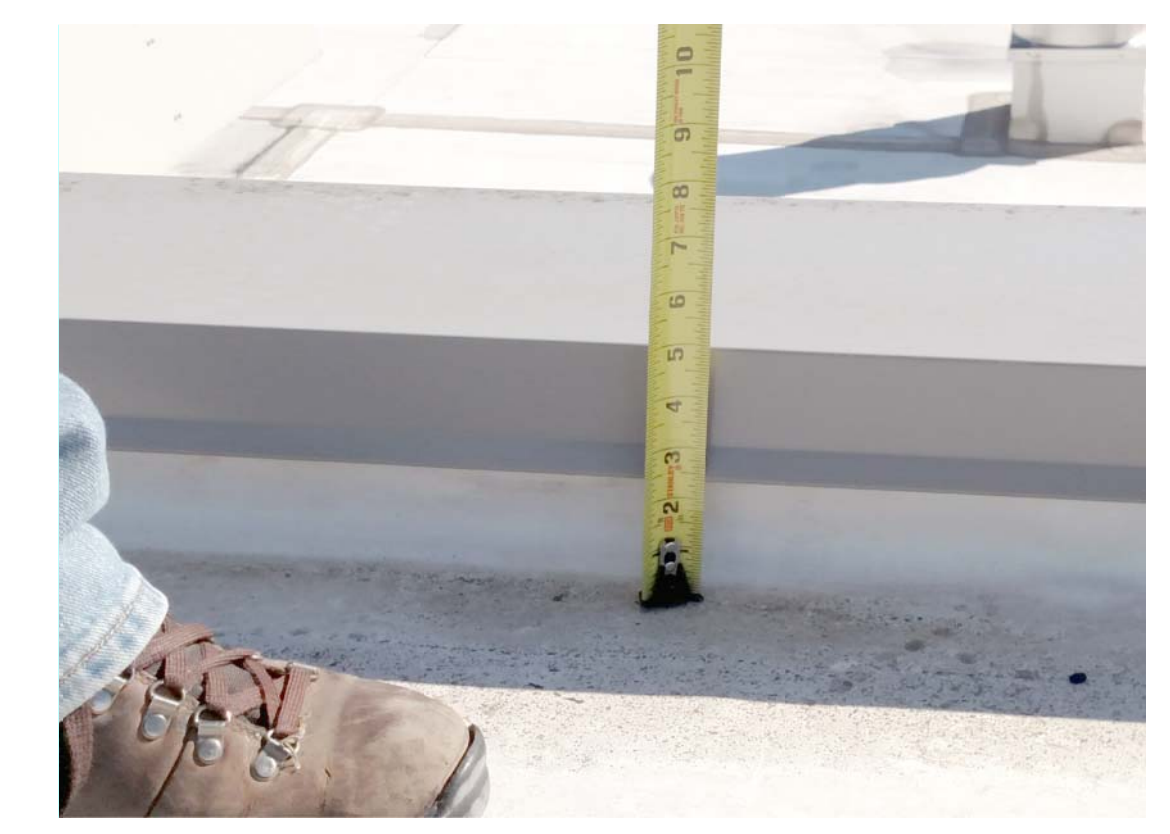
EXISTING CONDITION PHOTO 8 ROOF ACCESS LOCATION #2 SCALE: N.T.S.
