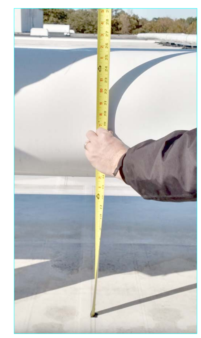
EXISTING CONDITION PHOTO 7 ROOF ACCESS LOCATION #6 SCALE: N.T.S.
