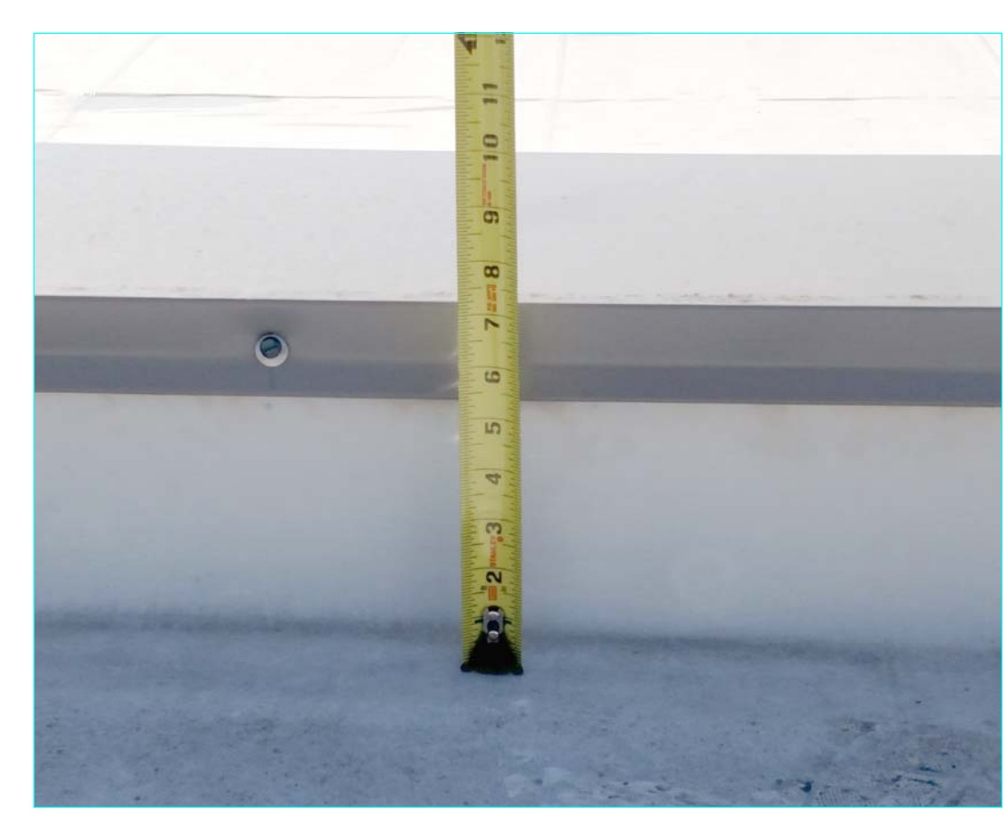
EXISTING CONDITION PHOTO 9 ROOF ACCESS LOCATION #3 SCALE: N.T.S.
