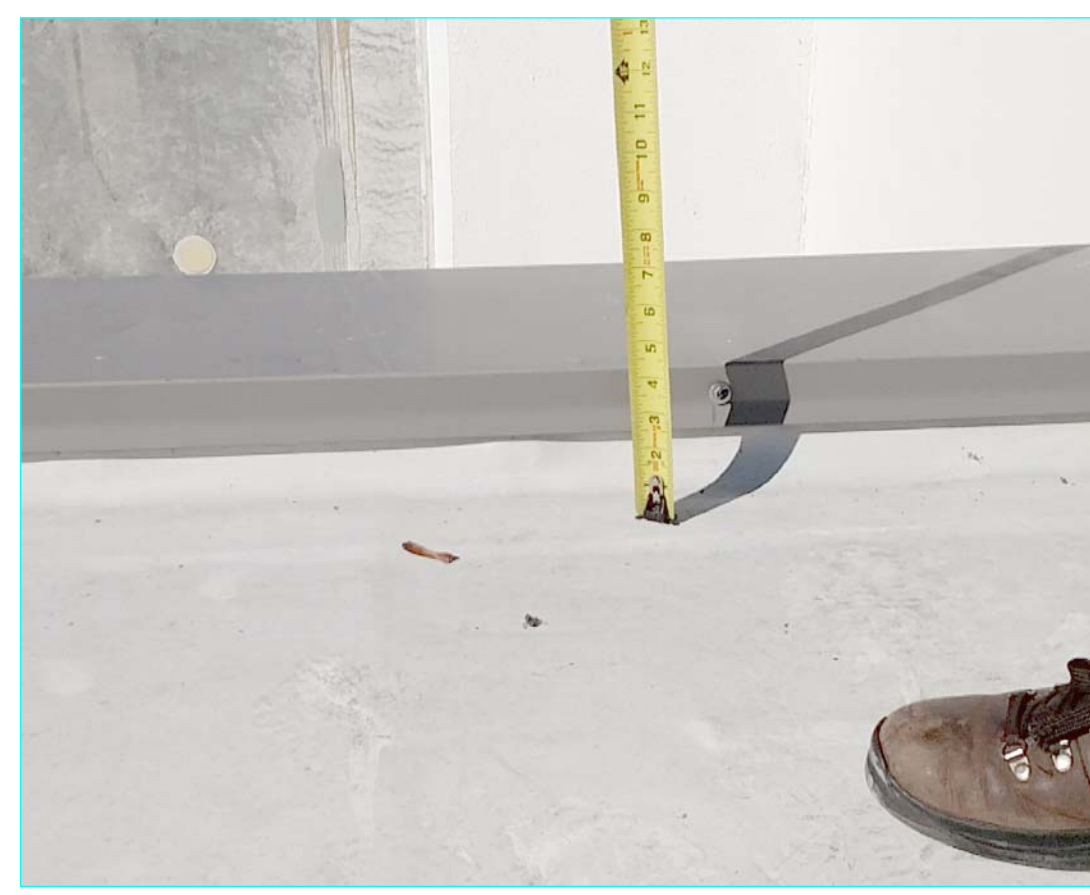
EXISTING CONDITION PHOTO 16 ROOF ACCESS LOCATION #4 SCALE: N.T.S.
